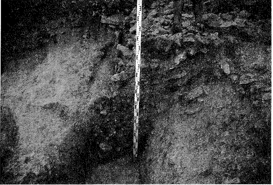
Fig. 6. Outer facing of the wall
