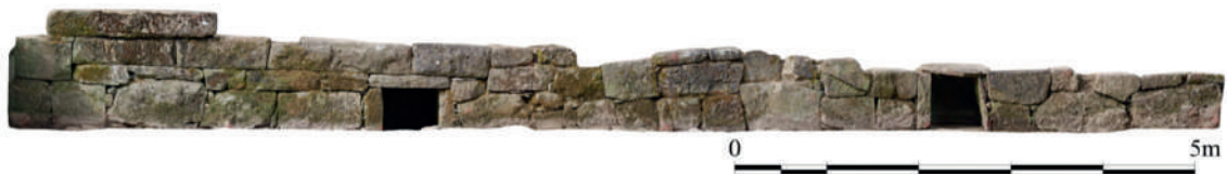
Fig. 6. Photogrammetry of the western wall where the niches are situated (compiled by B. Wojciechowski)
