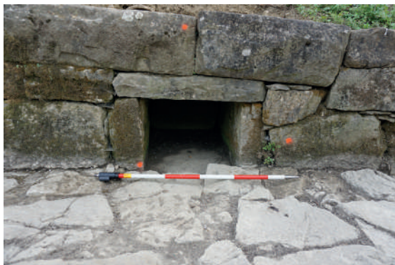
Fig. 7a. View of the southern niche (photo by M. Lemke)
