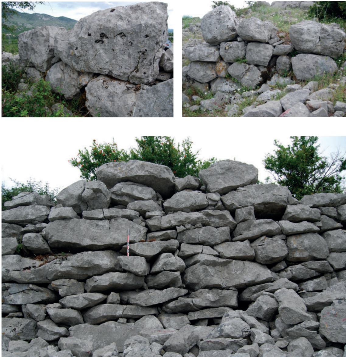
Fig. 14. Different techniques of the fortification wall at Vorfa (photo S. Shpuza)
