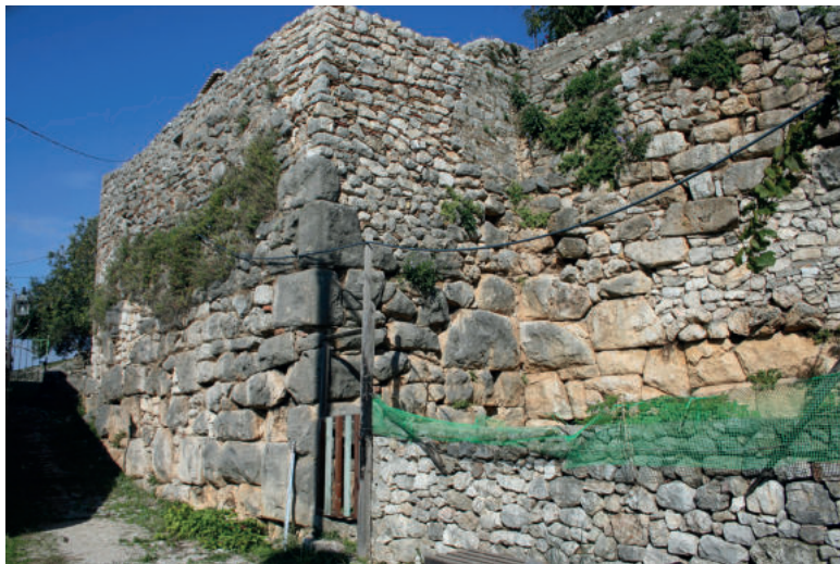
Fig. 7. View of the quadrilateral tower (photo K. Çipa)
