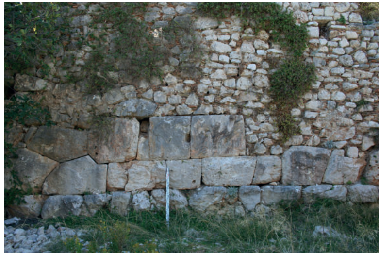
Fig. 4. View of the northern wall (photo K. Çipa)
