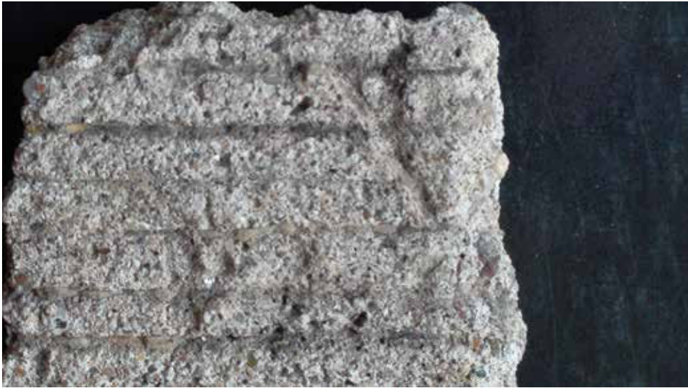
Fig. 12. Fragment of a wall “scratched” with a “like-a-comb” tool (photo P. Dyczek)
