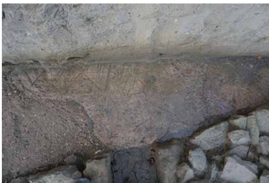
Fig. 32. Repairs to the floor of the bath (photo P. Dyczek)
